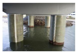
A three-year collaborative development project between Joinlox and USQ resulted in the development and commercialisation of a new type of composite pile repair system made of a prefabricated fibre-reinforced polymer (FRP) jacket with an innovative joining system for infrastructure rehabilitation.
