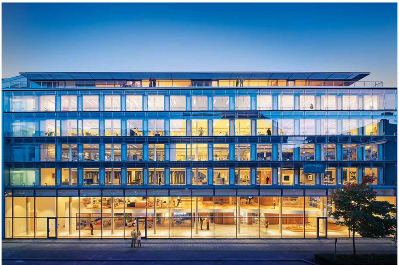
Steelcase Innovation Center Copyright: Steelcase
